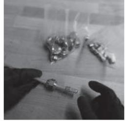
**3.** Hand tighten the IGLOO QUICK fitting without using tools. *Note:* Lubricating the contact surfaces of the 2 pieces of IGLOO QUICK fitting results in a stronger joint.
