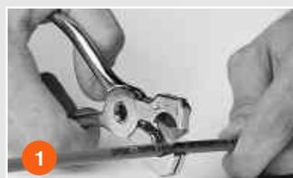
1 Cut the Quadra DN2 capillary hose to the required length using the special WXA004 cutter.
